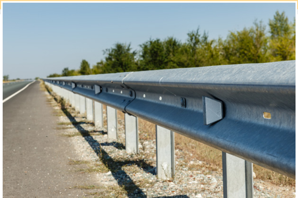
This photo shows a guardrail segment with reflectors, which demonstrates redundancy. The reflectors will help keep vehicles on the road, but if needed the guardrail will prevent vehicles from leaving the road.
