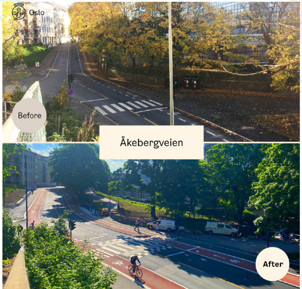
View of the street Åkebergveien in Oslo, Norway. Parking was removed to make room for a temporary bike lane going uphill before the street was rebuilt.
