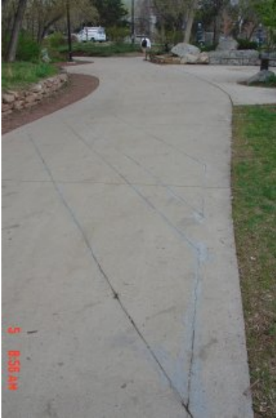
In-pavement loop detector for automated bicycle counts (Michael Gardner-Sweeney, City of Boulder, CO)
