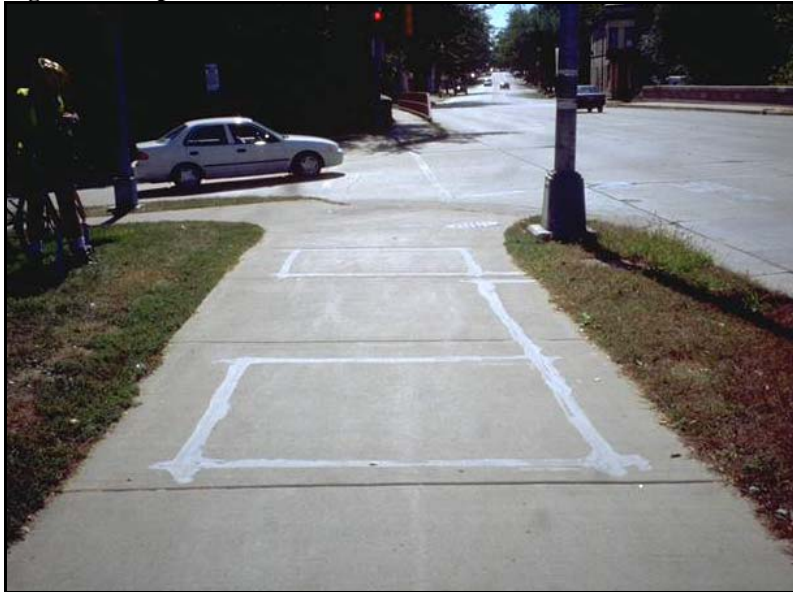
Figure 1. Loop Detector in Shared-Use Path Pavement
